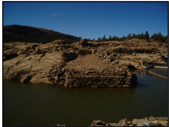
Alpine Highway bridge abutment. Photo by Frank Tortorich
