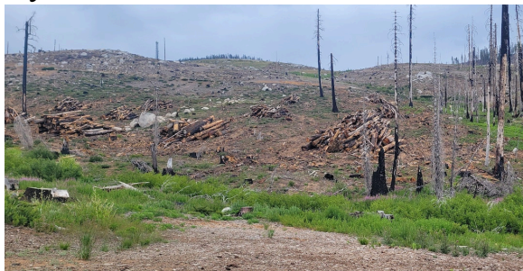
Cutting and piling of dead trees in preparation for burning piles and tree planting.
